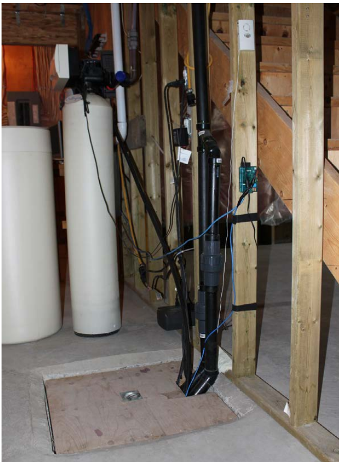
Figure 4. Finished Pit View
